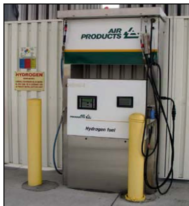
Figure 22. Compressed Hydrogen Dispenser
