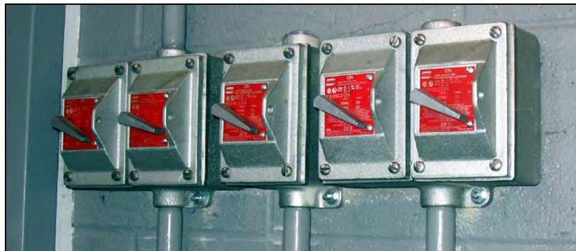
Figure 28. Explosion Proof Switches
