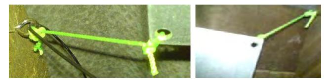
The plate is positioned between 3 and 3.5 metres (10 to 12 feet) above the ground and the attachment to the plate is also heavy-duty 8 swg cable:
