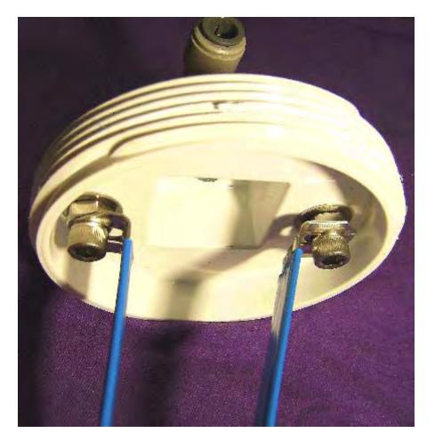
In order to ensure that the stainless steel straps are tightly connected to the electric wiring, the cap bolts are both located on the robust, horizontal surface of the cap, and clamped securely both inside and out. A rubber washer or rubber gasket is used to enhance the seal on the outside of the cap. If available, a steel washer with integral rubber facing can be used.
