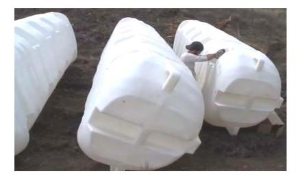
THE POSITIONING OF THE TANKS IS IMPORTANT AS THEY HAVE TO BE JUST BELOW THE ROOF SO THAT RAINWATER FLOWS INTO THEM UNDER GRAVITY AND YET THEY HAVE TO BE HIGHER THAN SHOWER-HEADS FOR THE SAME REASON (UNLESS A PUMP IS USED FOR SHOWERS). A SIMPLE FILTER IS USED TO REMOVE ANY BLOWN MATERIAL WHICH FINDS ITS WAY INTO THE WATER INTAKE.
