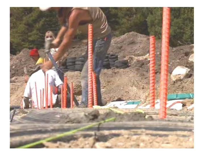
STEEL BARS CALLED "REBAR" ARE DRIVEN INTO THE WALLS AND POSITIONED TO THE EXACT HEIGHT AND THEN A REINFORCED CONCRETE RING IS CAST AROUND THE TOP OF THE WALLS TO GIVE OVERALL STRENGTH TO THE STRUCTURE BEFORE THE VERY HEAVY TREE TRUNKS ARE PLACED ON IT.
