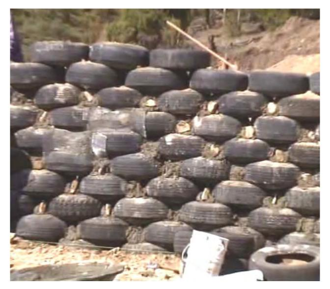
THE TYRES ARE OVERLAPPED IN SUCCESSIVE ROWS, FORMING A STABLE STRUCTURE, AND THEN MORTAR GROUTING IS APPLIED BETWEEN THEM. THE OUTSIDE IS ENCLOSED IN AN EARTH BANK AND THE INSIDE IS SMOOTHED OVER.
