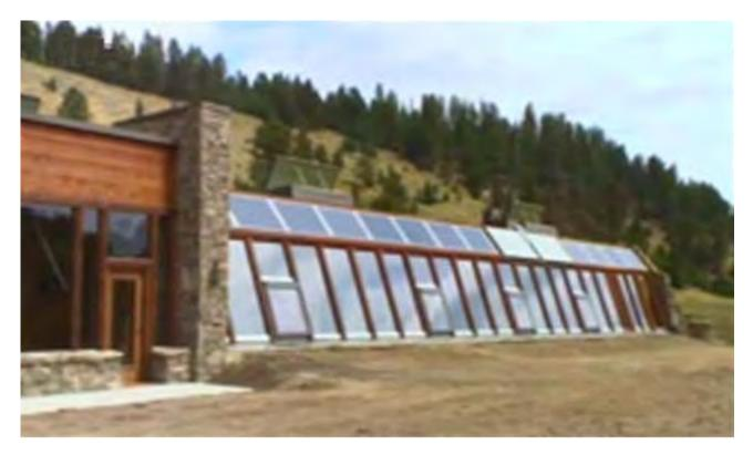
THE WALLS OF THE PROPERTY ARE SEVEN FEET (2.13 METRES) THICK. THIS IS TO ALLOW THE USE OF FAIRLY SIMPLE MATERIALS AND MORE IMPORTANTLY, TO PROVIDE THERMAL MASS WHICH KEEPS THE INSIDE OF THE BUILDING WARM IN WINTER AND COOL IN SUMMER. THERE ARE NO SIGNIFICANT BILLS FOR HEATING OR COOLING AND NORMAL ELECTRICAL EQUIPMENT IS RUN FROM THE POWER PROVIDED BY THE SOLAR PANELS, A BANK BATTERIES AND A MAINS INVERTER.
