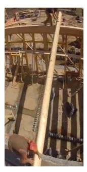
THESE BEAMS ARE VERY HEAVY AND ARE QUITE CAPABLE OF CAUSING SERIOUS INJURY IF NOT HANDLED CAREFULLY AND SENSIBLY. THEY FORM THE JOISTS WHICH SUPPORT THE ROOF AND AS THERE IS A GAP OF ONLY ONE FOOT BETWEEN THEM, MANY ARE NEEDED. THEY ARE ATTACHED TO THE TOP OF THE WALL BY STEEL RODS DRIVEN THROUGH THEM AND INTO THE TOP OF THE WALL.
