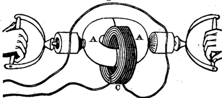
to separate them. The handles are attached to the armatures by ball and socket joints, to prevent them from being twisted or wrenched by irregular pulling. The induction of magnetism in these armatures by means of the current from a thermo-electric battery has already been mentioned in § 56.
